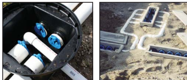
Custom Distribution Boxes with Equalizers installed
